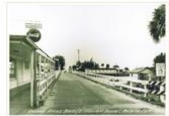
IR13 bridge with store.jpg
